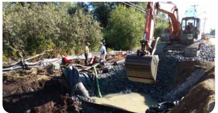
Above: Excavating wetland peat. Below: Adding rock fill.
