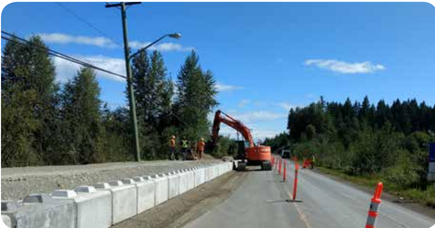
New lock block retention wall installed.
