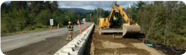
Levelling pre-load gravel along wetland.
