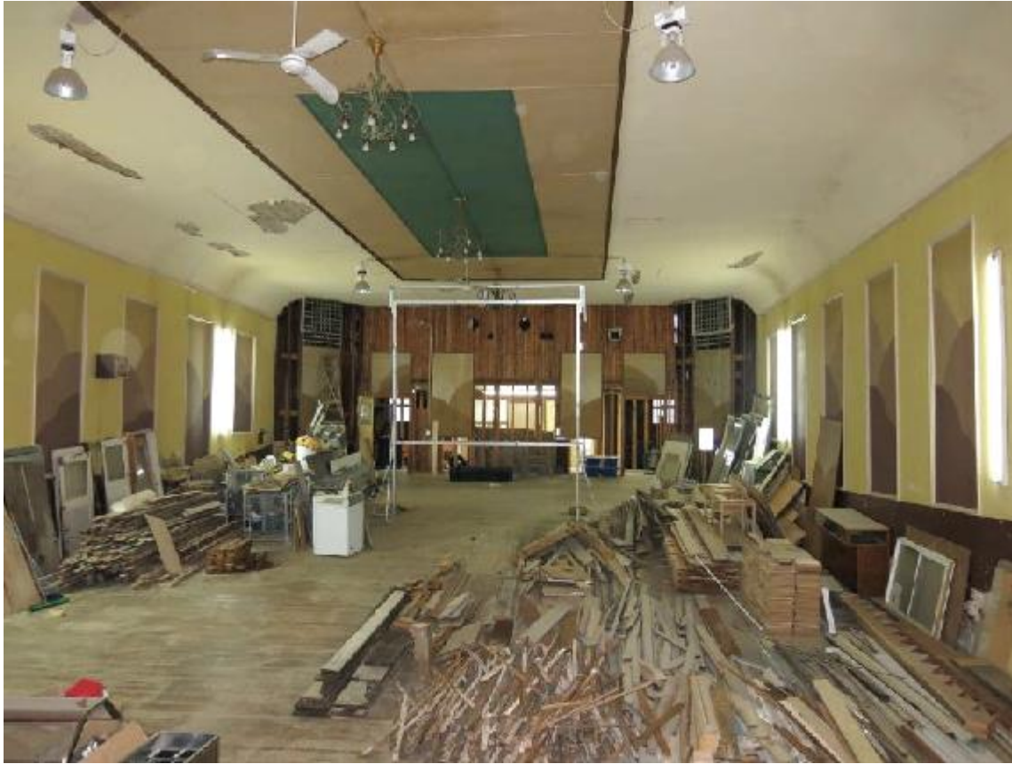
Theatre auditorium looking towards entrance
