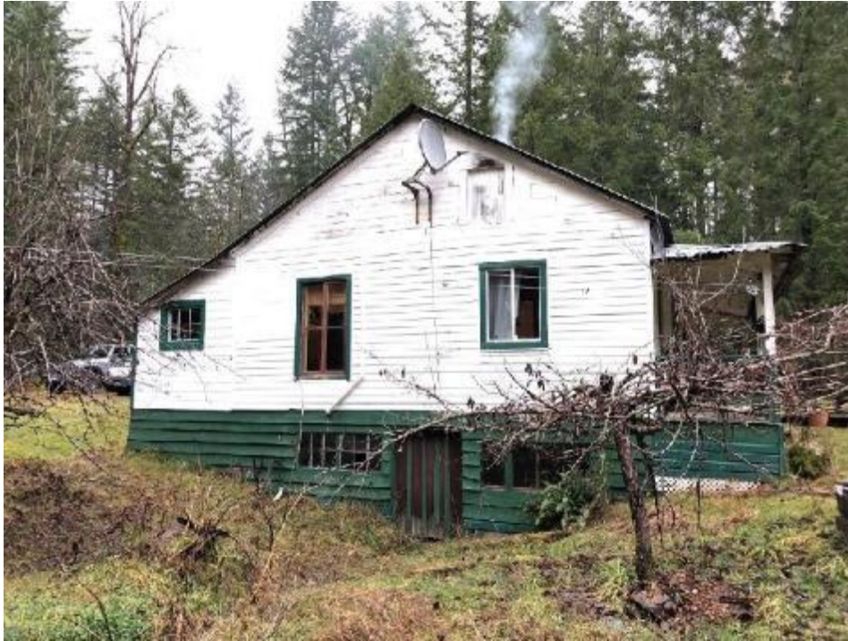
Side view - west Creek bed
