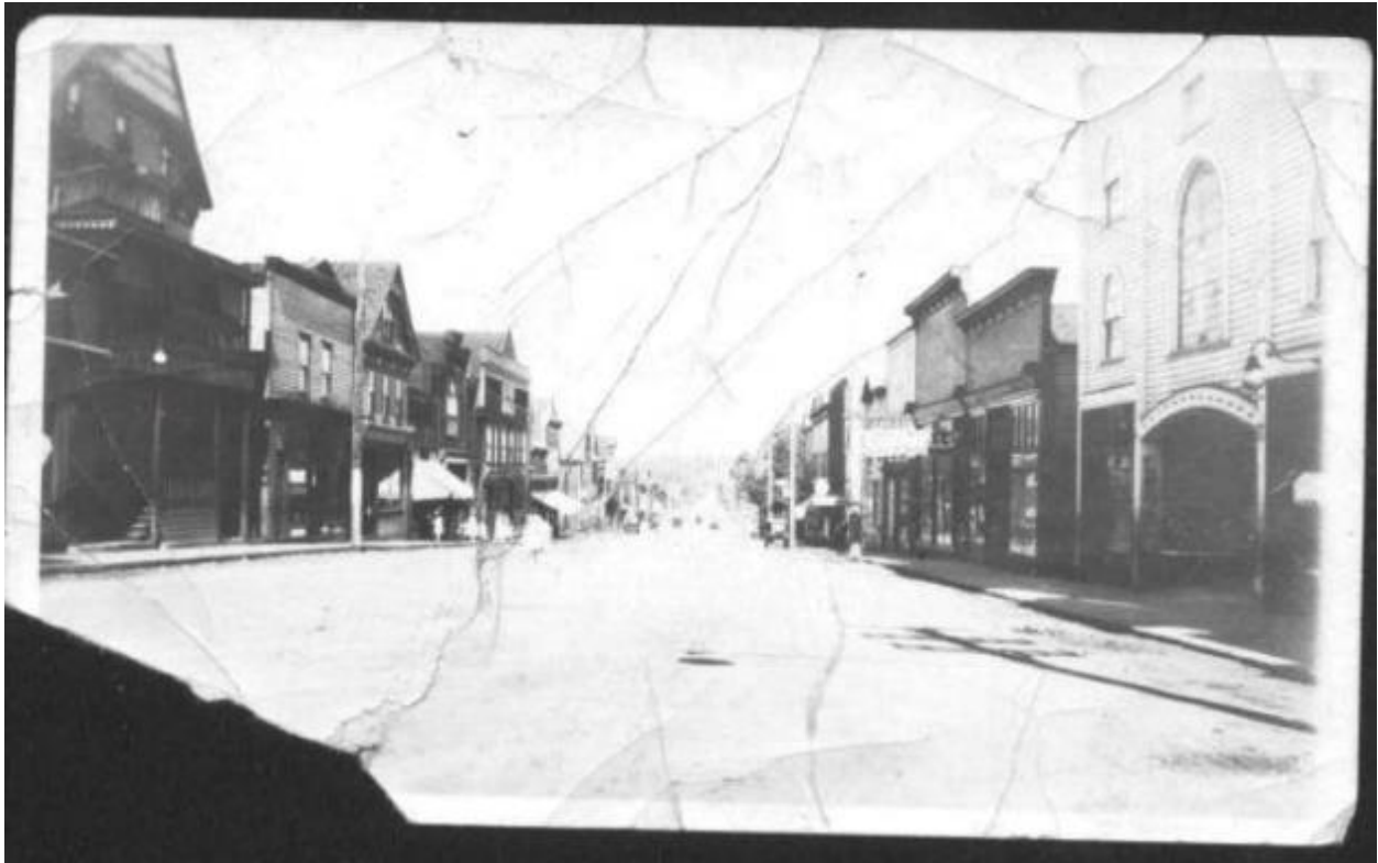
The 1914 wood clad Ilo-Ilo Theatre with arched entrance - which was destroyed by fire in 1932, is the
