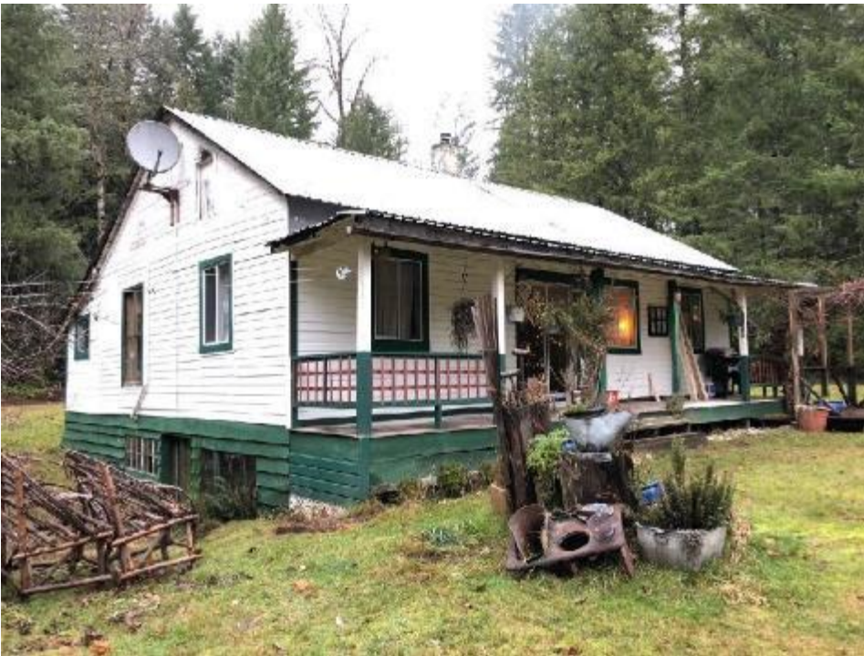
Rear view from southwest corner
