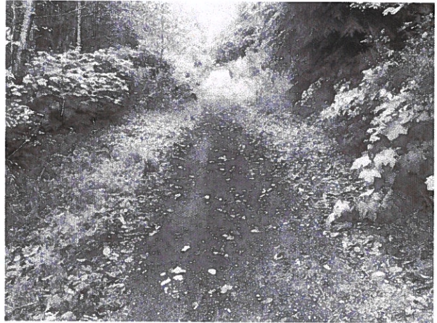
Photo 14: View of rail grade trail in the area that the orange stormwater would cross if there was a defined crossing. No waterway was located.
