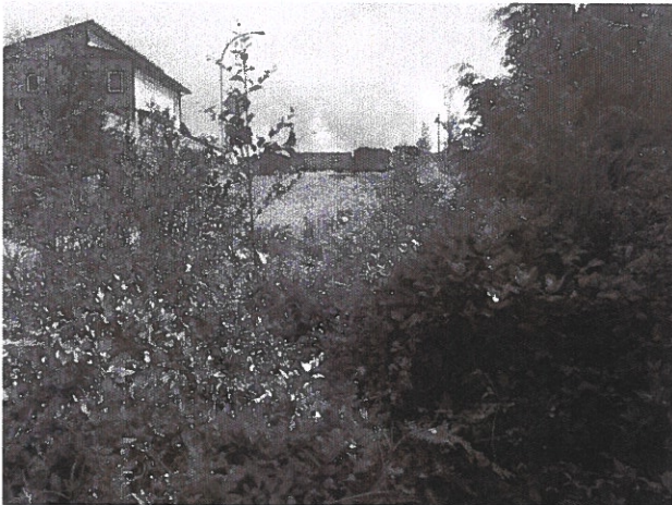
Photo 3: View of existing overland stormwater outlet location at end of Solport Street. There is a band of terrestrial vegetation including salal between the outfall and the low lying area.
