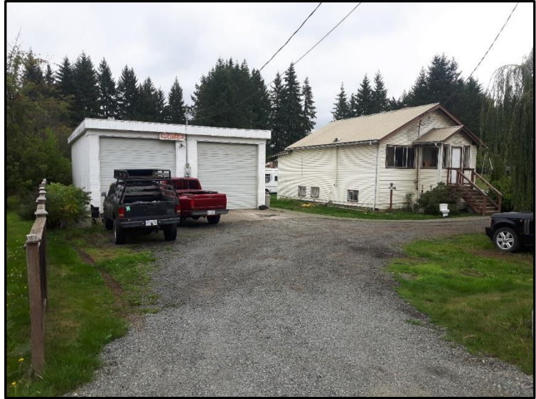
Figure 2: View of the Property from Cumberland Road
