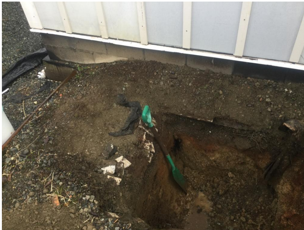
Photo 4: Test pit 2 on neighbour's side of building
