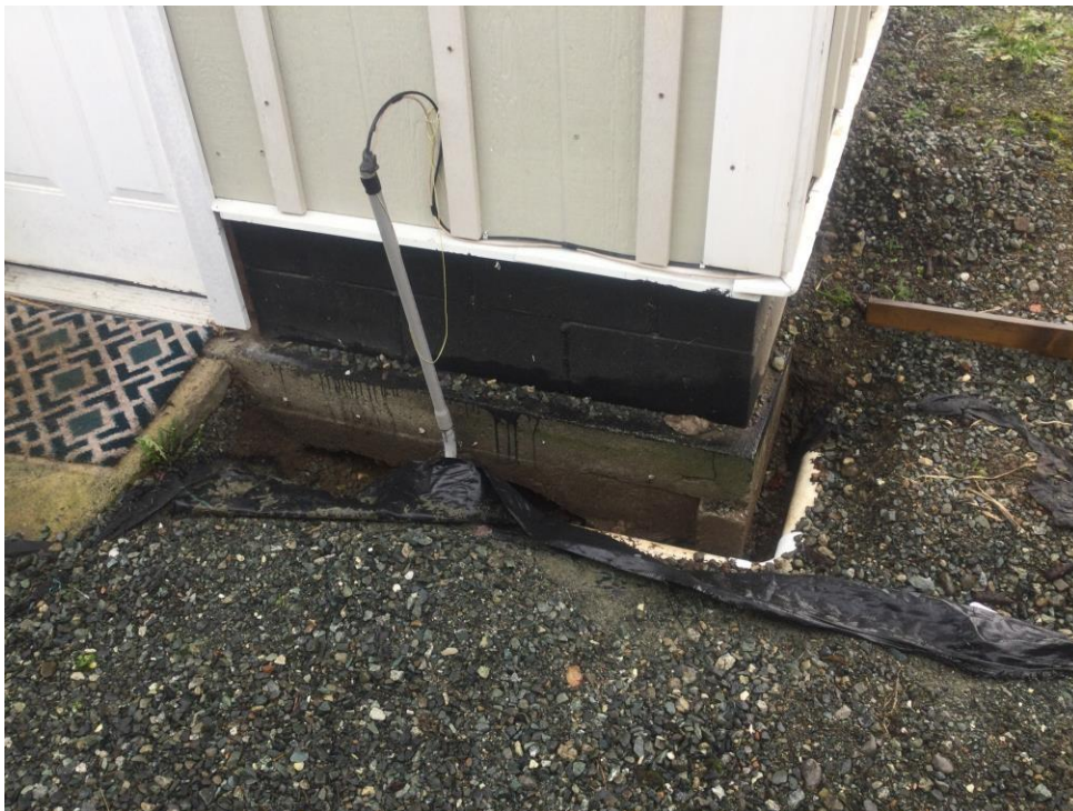
Photo 2: Existing Slab-on-Grade foundation with cinder block frost wall.
