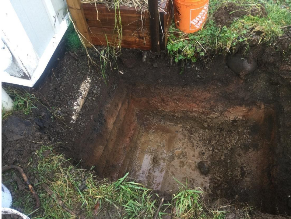
Photo 3: Test pit 1 on alley side showing perimeter drain.
