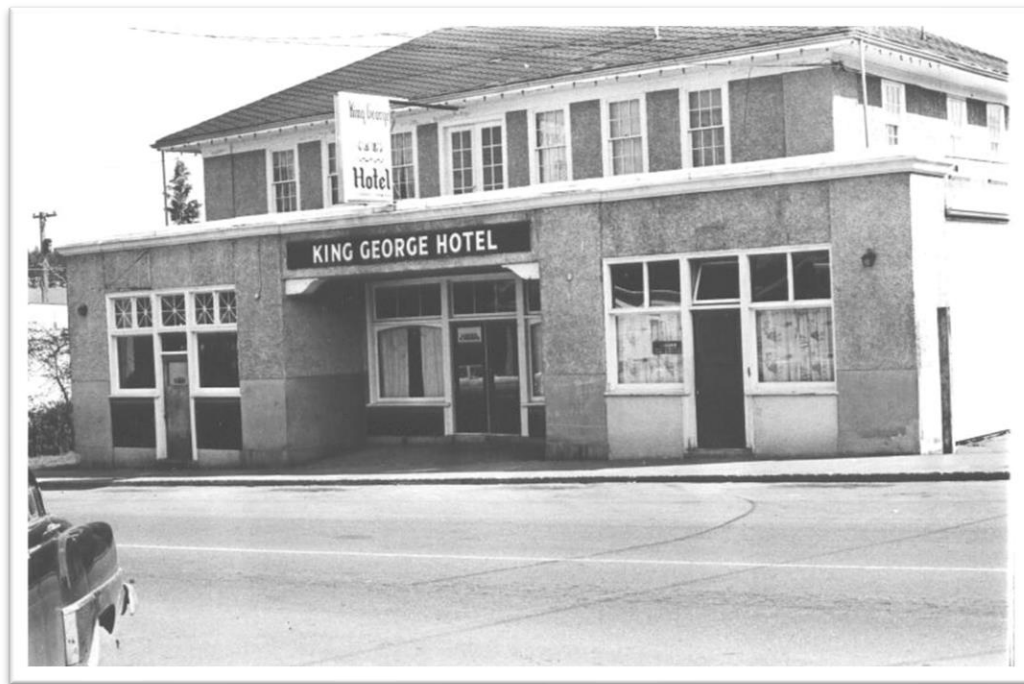
Figure 18: King George hotel after 1933 sign on left of hotel states government liquor store, c.1950s Source: Cumberland Museum Archives (C030-157)
