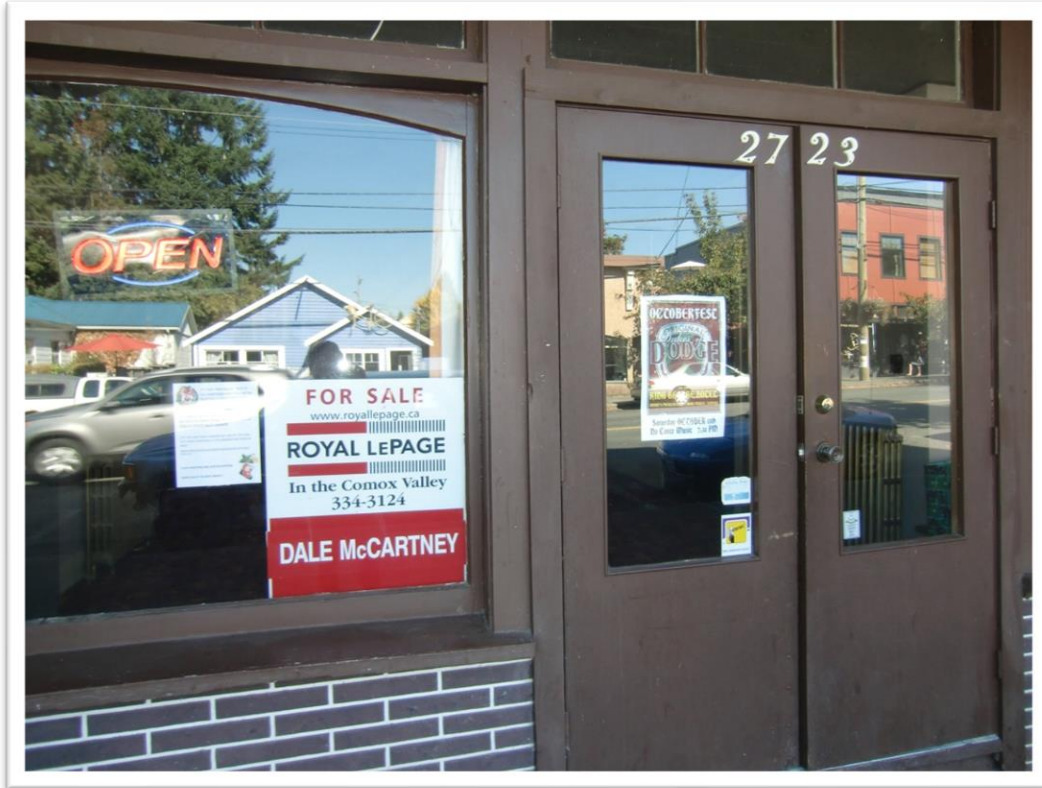
Figure 6: Current entrance of the Hotel
