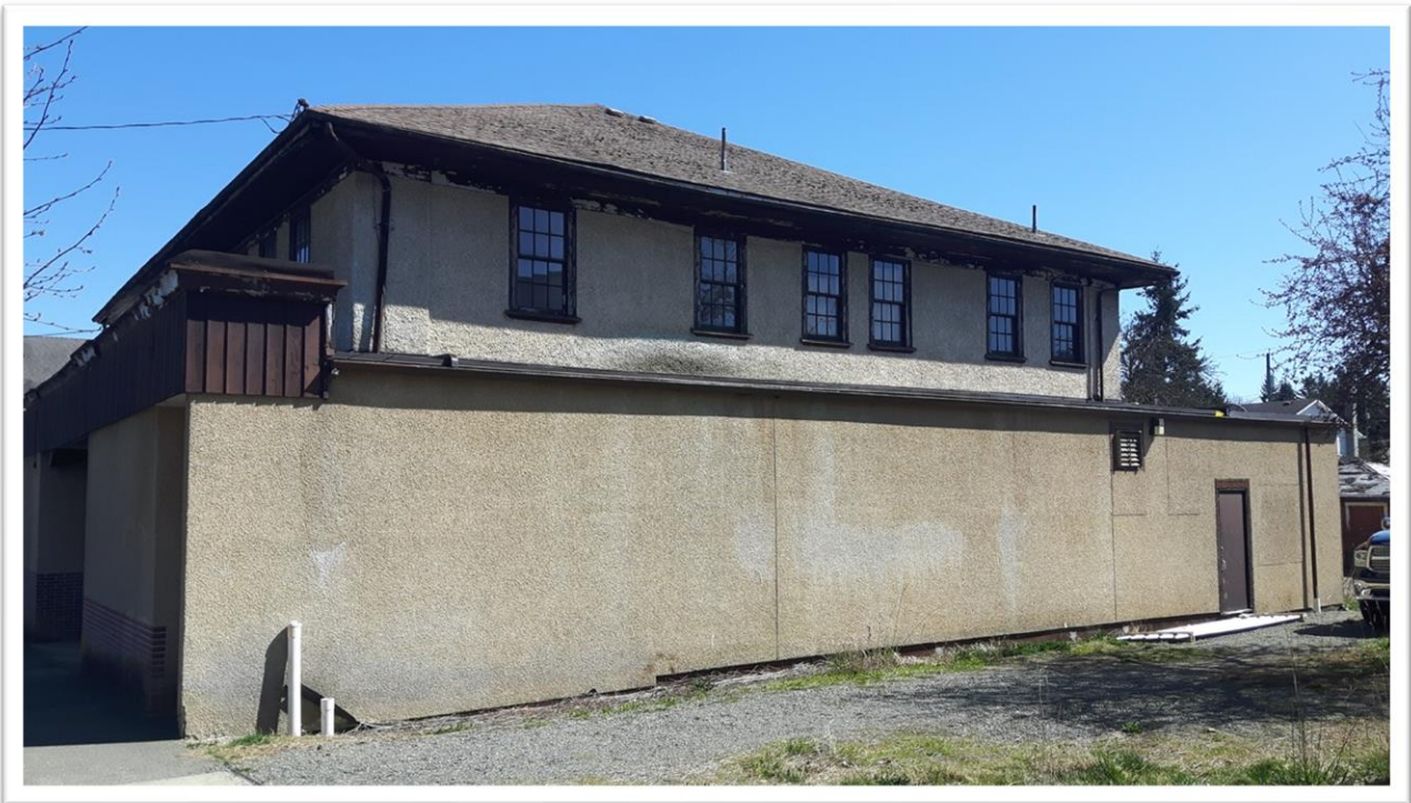
Figure 5: West side view of the King George Hotel, April 2021
