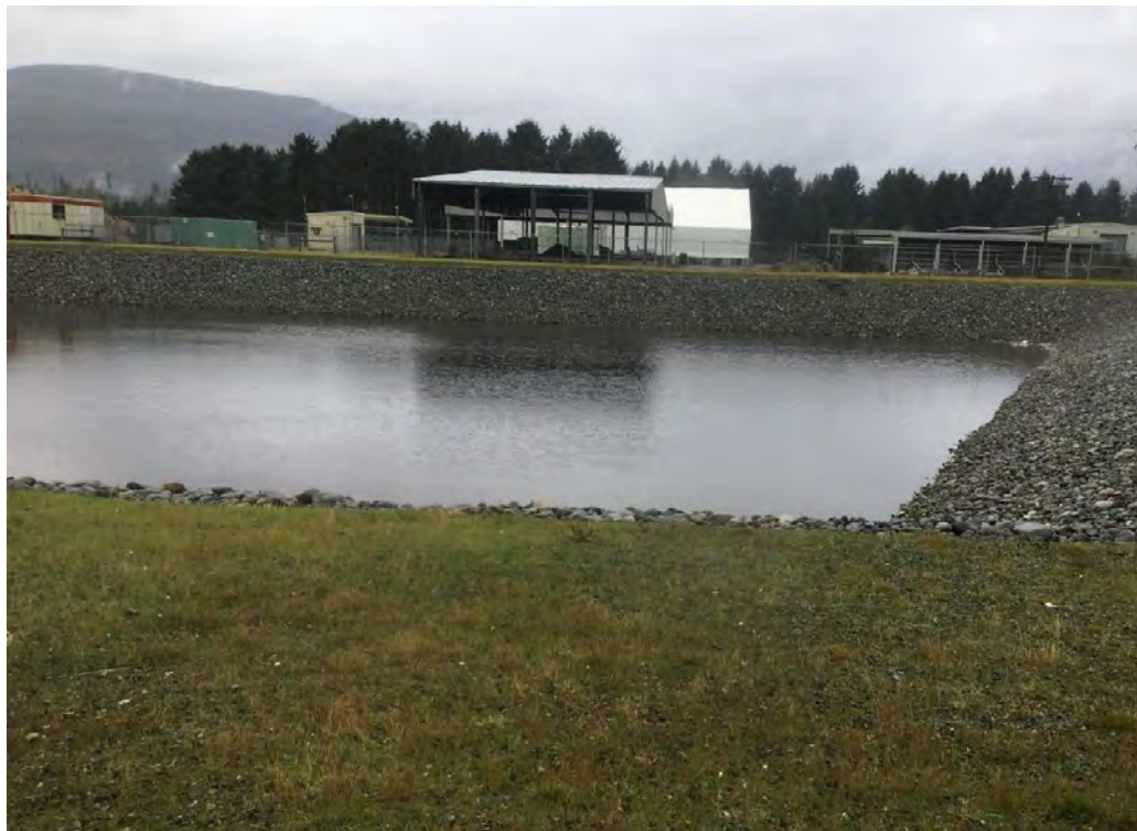
Photo 8. Existing leachate pond #1.
