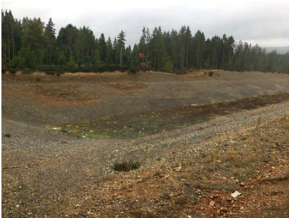
Photo 6. Looking southwest at the existing stormwater pond.
