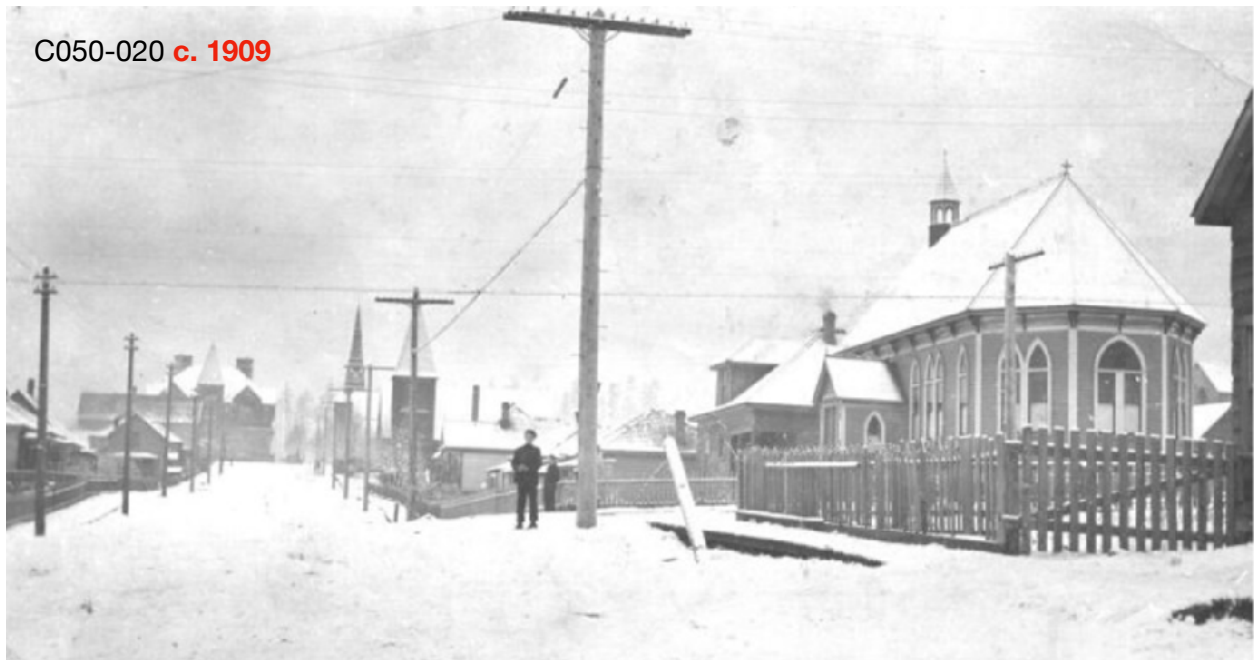
Penrith Avenue in 1909 soon after the manse was built next door but the bell tower not yet erected.
