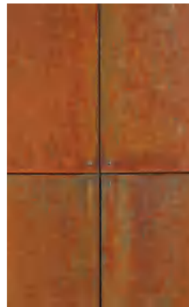
CORTEN STEEL PANEL, NON-COMBUSTIBLE
