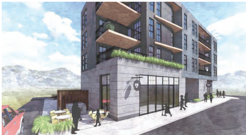
VIEW OF CRU 3 PATIO ON 2ND STREET
