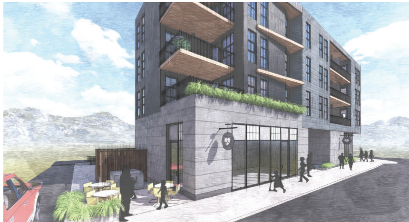
VIEW OF CRU 3 PATIO ON 2ND STREET
