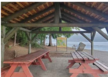
Repaired picnic shelter at beach
