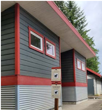
New washroom and shower building
