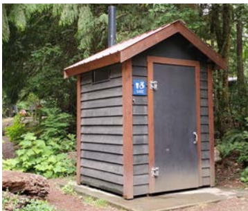
New vault toilets (pit toilets removed)
