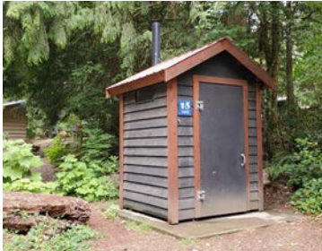
Existing: Park vault toilet installed by the boat ramp.
