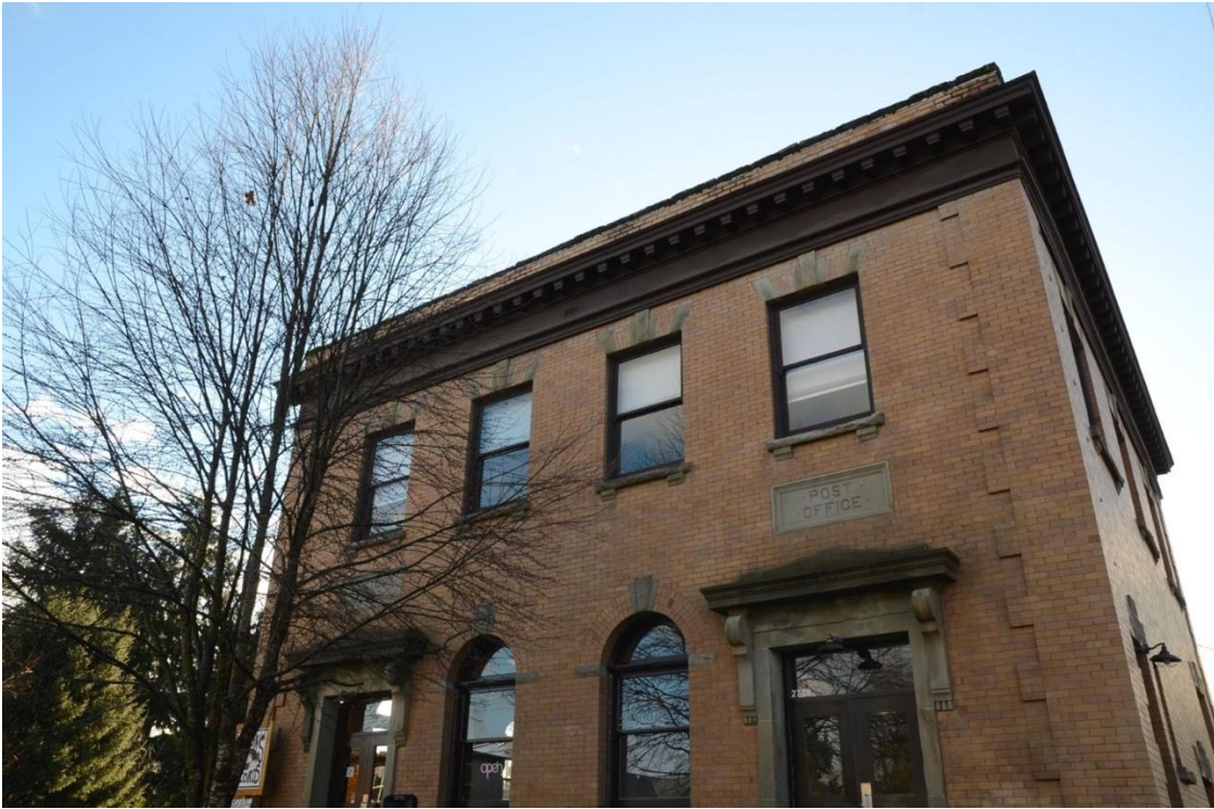
Figure 19: The Old Post Office building on Dunsmuir Avenue.
