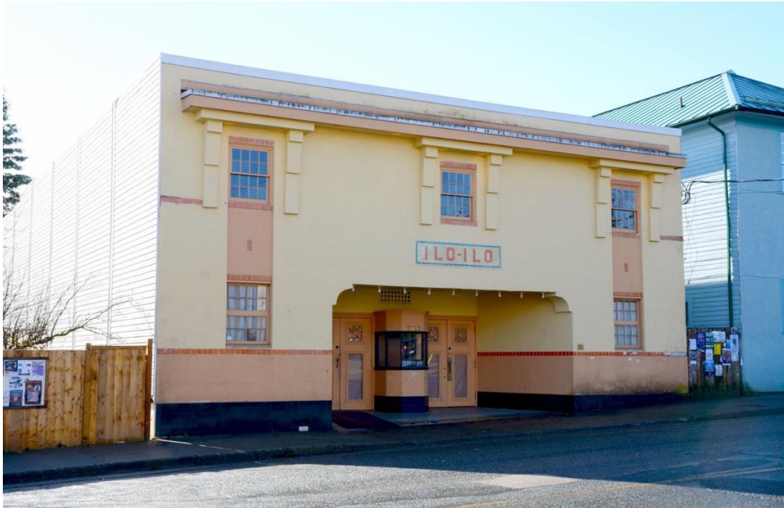
Figure 2: A unique Art Deco building, the Ilo Ilo Theatre on Dunsmuir avenue.
