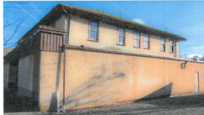
WEST SIDE OF BUILDING
