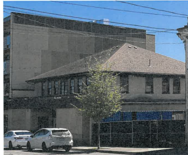
DUNSMUIR - LOOKING EAST
