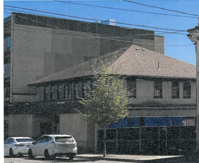
DUNSMUIR - LOOKING EAST
