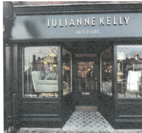
FRONT FACADE WOOD PANELLING & TRIM - SHERWIN WILLIAMS "IRON ORE"
