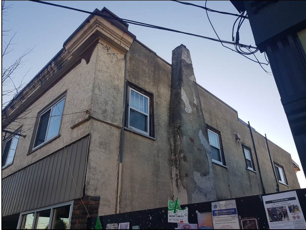
side view (west elevation)
