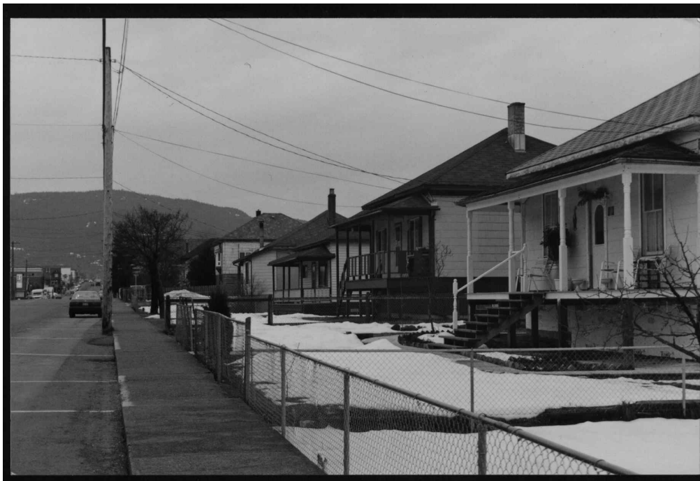
Photograph of the Bevan Houses at 2814, 2818, 2822, and 2824 Dunsmuir Avenue, 1997. Source: Cumberland Museum & Archives, C270-015.
