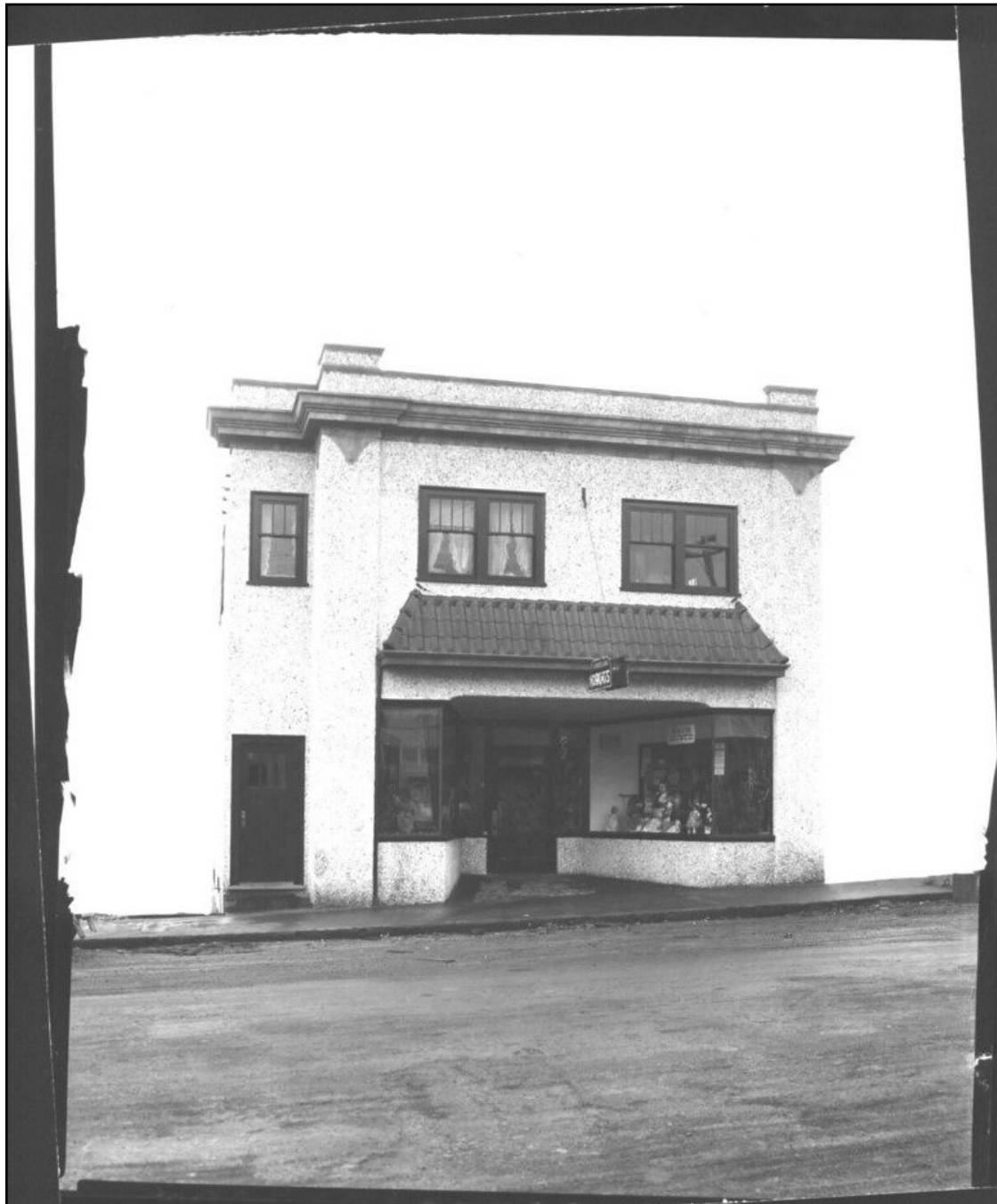
Photograph of Cumberland Drug Store. The photograph shows the building with its original recessed entry, storefront windows, stucco cladding at ground floor and tiled canopy. Source: Cumberland Museum & Archives, 2719 Dunsmuir Avenue – Building file, year unknown.
