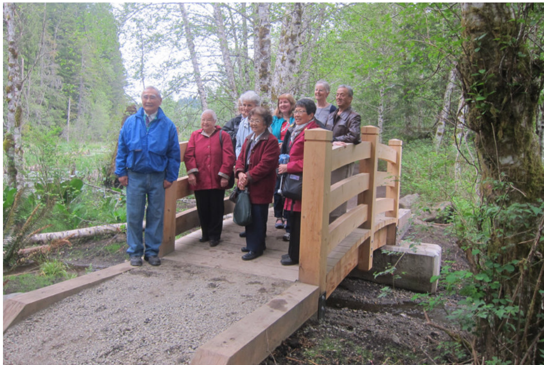
Bridge installed in 2013 on the Wellington Colliery Railroad trail over Perseverance Creek
