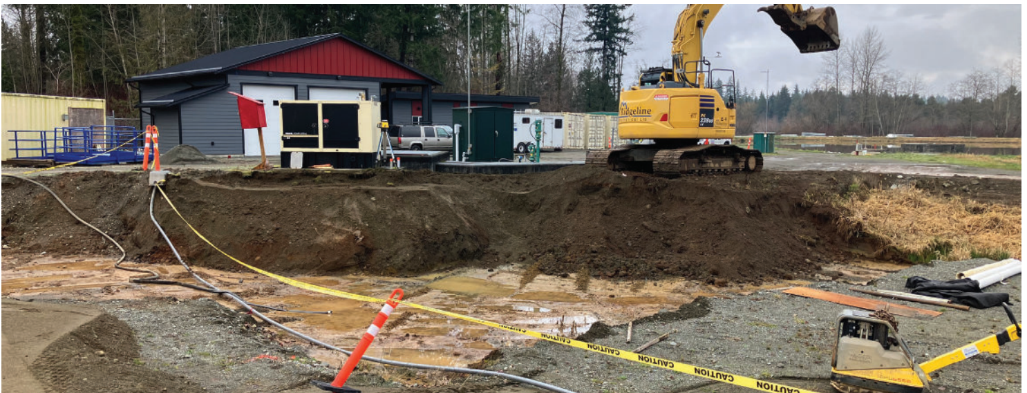
Headworks subgrade: Machines prepare the ground at the new site of the headworks. The new operational building, completed in late 2024, can be seen in background.
