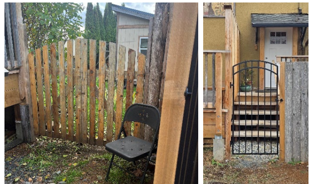
Wooden picket gate and Black metal gate as installed
