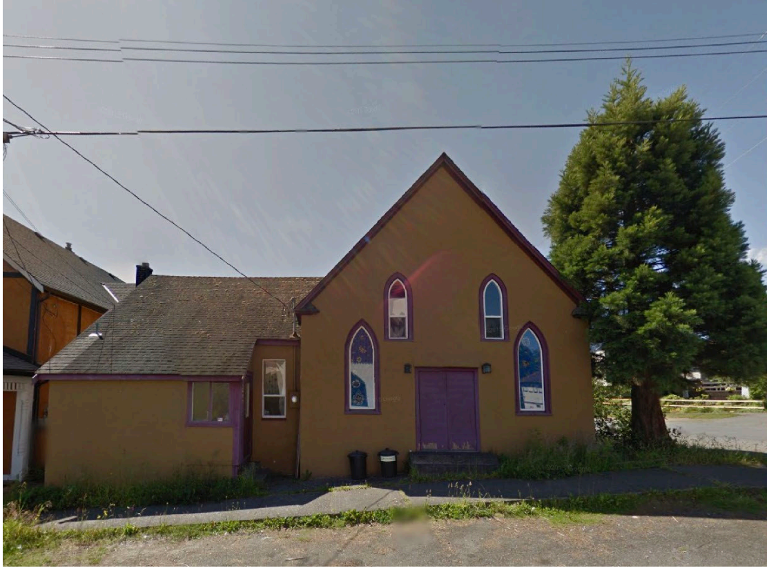
Front view (Penrith Ave)
