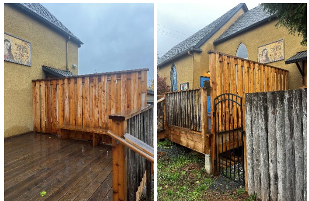
Divider, wooden fence and metal gate as installed
