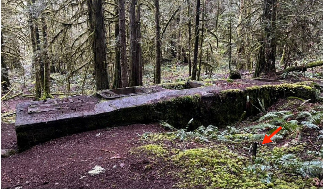
Above: View of the concrete structure from the rear (mountain side). The right portion of the structure appears to have been added. It is lower and has a smaller turbine pier and a smaller arched outlaw opening. Also visible (marked with an arrow) is the grounding rod.
