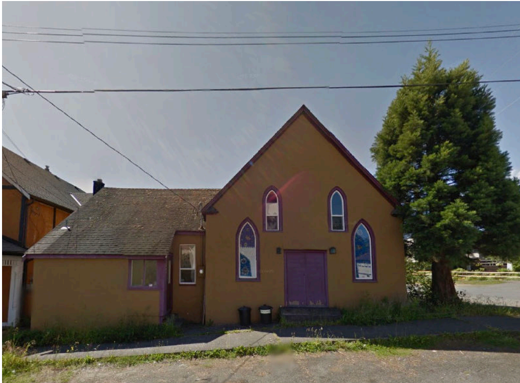
Front view (Penrith Ave)
