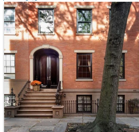
Figure 12-17: Example of prominent building entrance (guideline 14 e)
