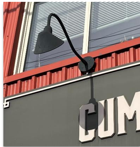
Figure 12-15: Example of sign illumination (guideline 13 e)
