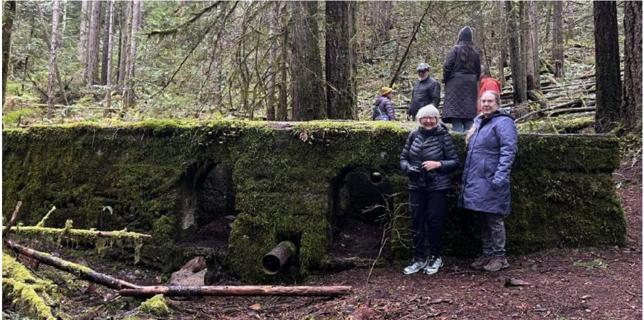
Above: View of the concrete structure (the elevation facing Chinatown) with two of the arched water outflow openings as well as the outflow metal pipe. Below: View of the top of the structure with embedded and bolted metal mounting plates, as well as the metal plate for anchoring the transformer.
