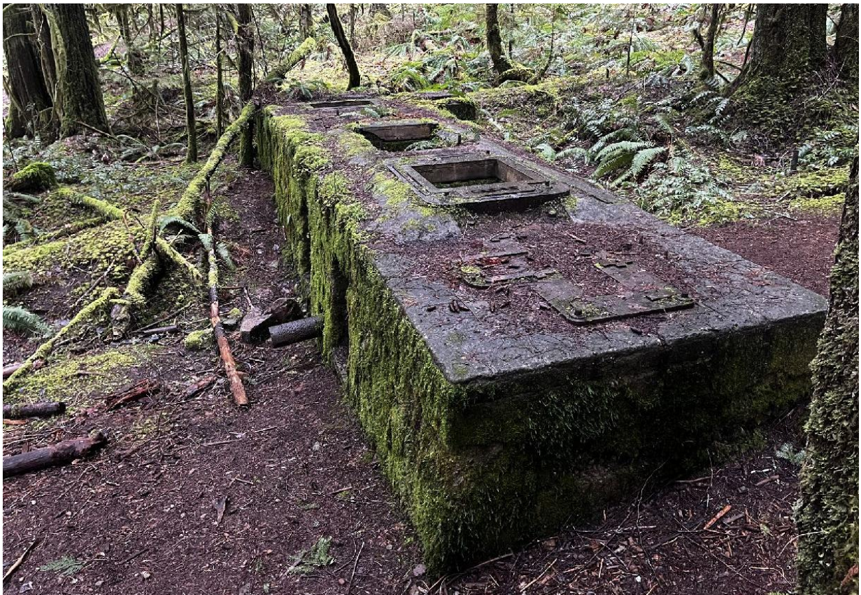
Above: View of the concrete structure (the elevation facing Chinatown) with two of the arched water outflow openings as well as the outflow metal pipe. Below: View of the top of the structure with embedded and bolted metal mounting plates, as well as the metal plate for anchoring the transformer.
