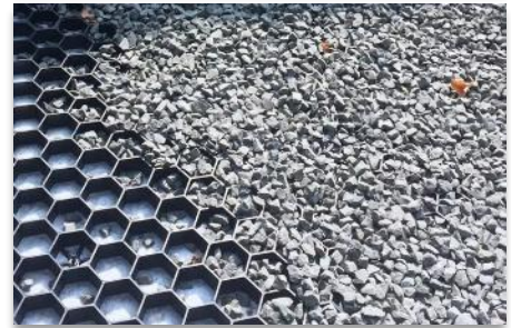
Figure 11.10-15: Example of permeable paving surfaces (guideline 6g)
