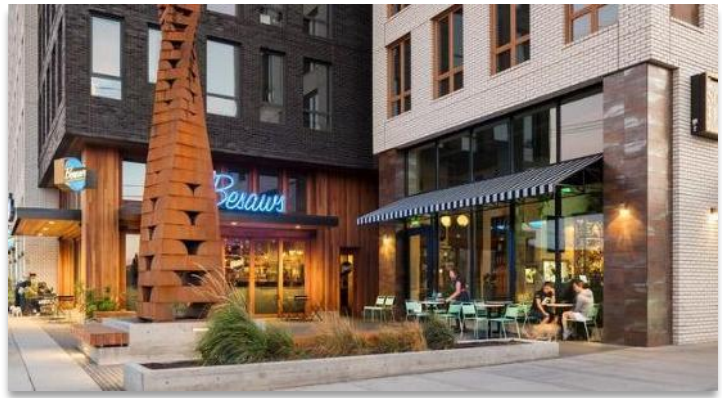
Figure 11.10-8: Example of ground floor commercial use oriented towards the public realm (guideline 3. o.)
