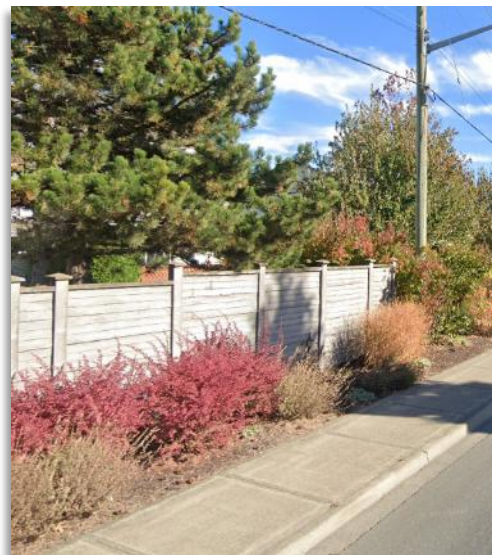
Figure 11.9-3: Example of sound attenuating fencing with a vegetative buffer in front (guideline 2l)
