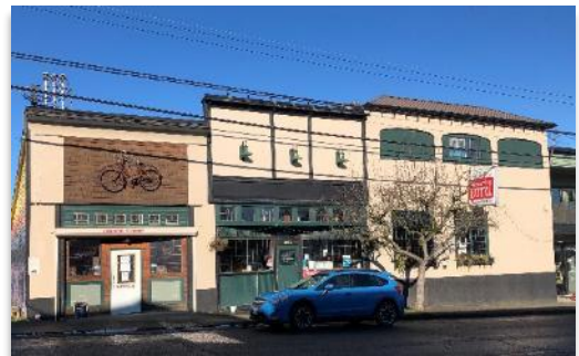
Figure 11.13-2: Examples of false front (top and middle), canted storefront entrance with transom windows (all), pitched roof (middle), hip roof (right -most building in bottom photo).
