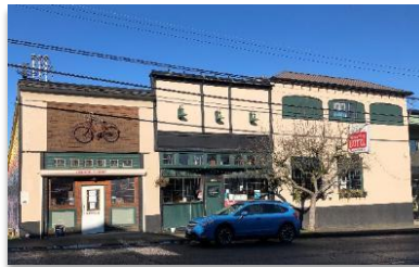
Figure 11.13-2: Examples of false front (top and middle), canted storefront entrance with transom windows (all), pitched roof (middle), hip roof (right -most building in bottom photo).
