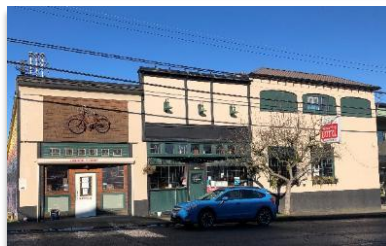
Figure 11.13-2: Examples of false front (top and middle), canted storefront entrance with transom windows (all), pitched roof (middle), hip roof (right -most building in bottom photo).
