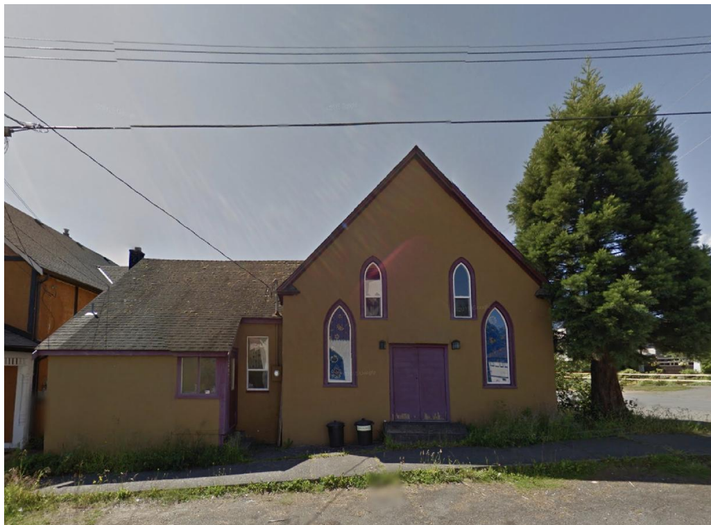
Front view (Penrith Ave)
