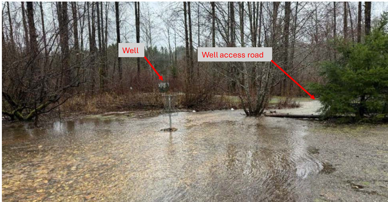
Figure 1.3 Looking downstream along avulsion channel in disc golf course on February 1, 2026, showing groundwater drinking water supply well and flooded access road for it. Photo courtesy of Adam Silverstein.
