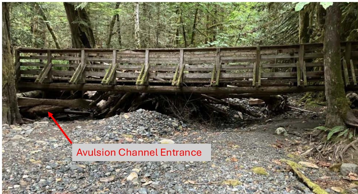
Figure 3.6 Looking upstream at the downstream side of trail bridge. Log jam on upstream side of bridge. Avulsion channel entrance as annotated. Photo taken July 16, 2026.
