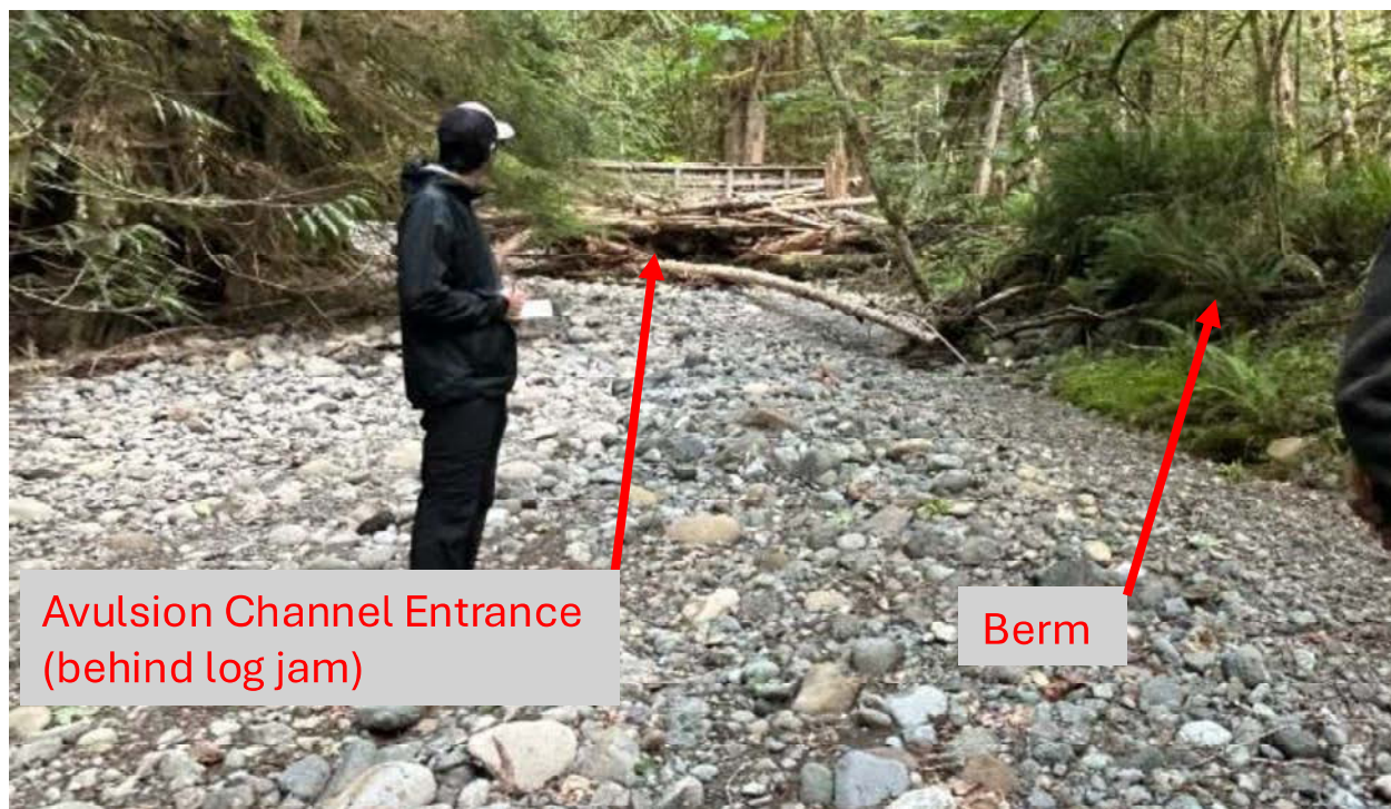
Figure 3.7 Looking downstream at trail bridge and log jam accumulated on it. Photo taken June 10, 2026.
